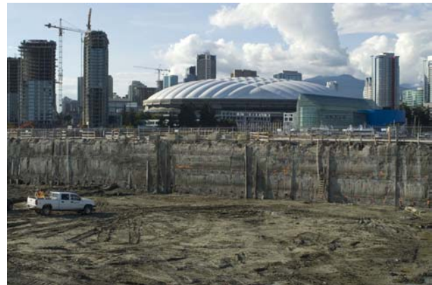
Photo 12- Excavated and trimmed jet-grouted wall
