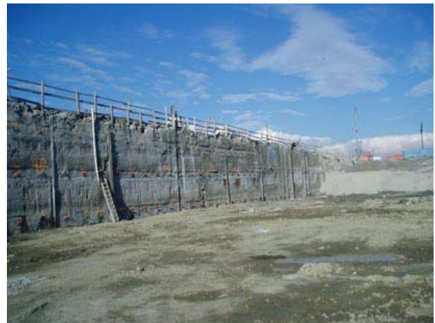
Photo 11- Excavated and trimmed jet-grouted wall
