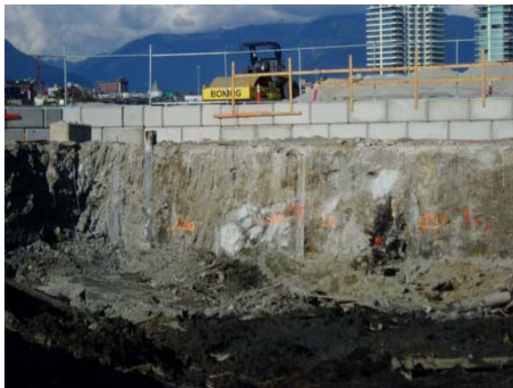
Photo 8 – Parcel 4 East Wall- Boulders
