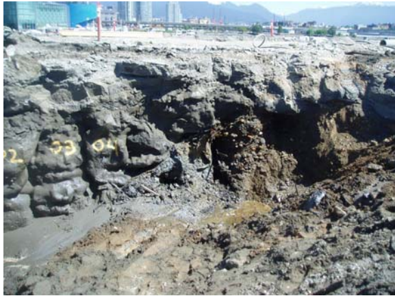
Photo 7– Parcel 4 detail of Photo 6
